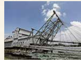
TANJUNG TUALANG TIN DREDGE NO. 5 - TT5
